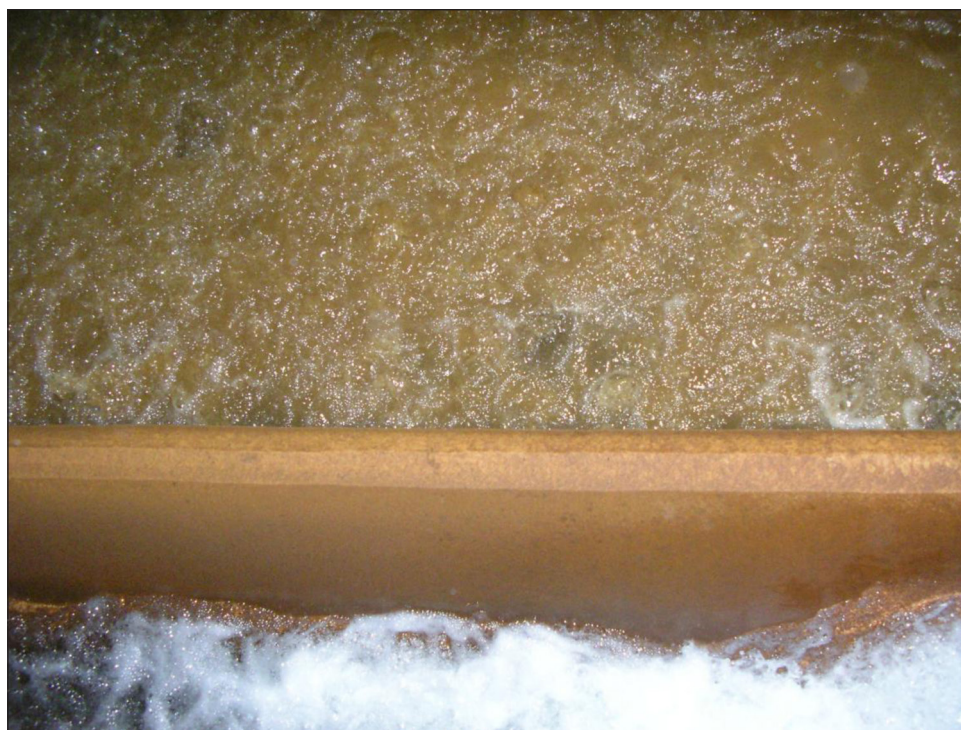
Fig. 1. Liquid backwash residual on the top of open gravitational filter (Antaviliai, Lithuania)
